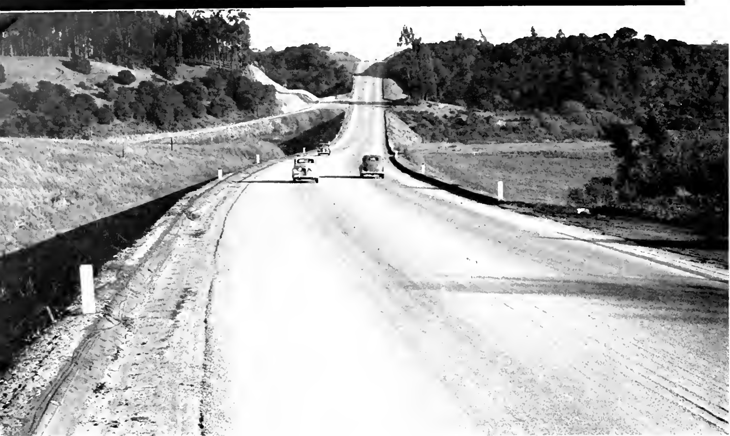
This stretch of new Watsonville-Rob Roy highway shows easy grade alignment and sight distance advantages.
